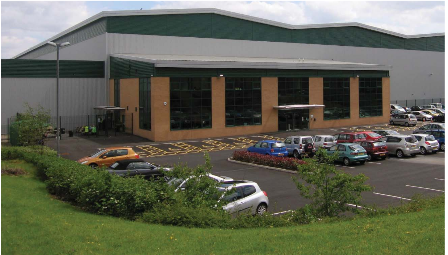
Tesco Distribution Unit, Bolton
